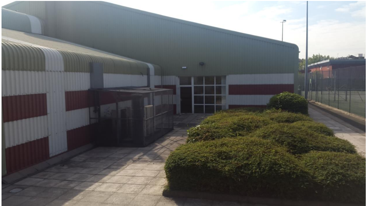
Image 2: Site of extension
